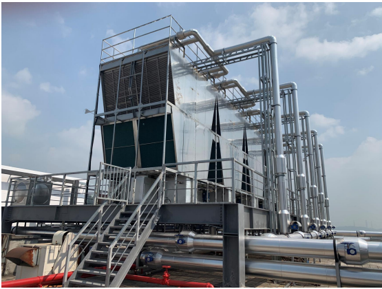
图 3 露点型间接蒸发冷却塔 Fig.3 Dew point type indirect evaporation cooling tower physical picture
